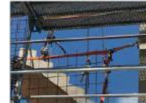
Positioning work with dynamic loads
