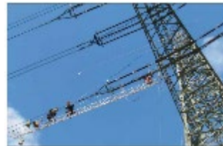
Overhead line construction
