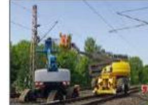
Construction of contact lines
